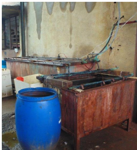
Before: Operation of process tanks without any timer and buzzer installed
